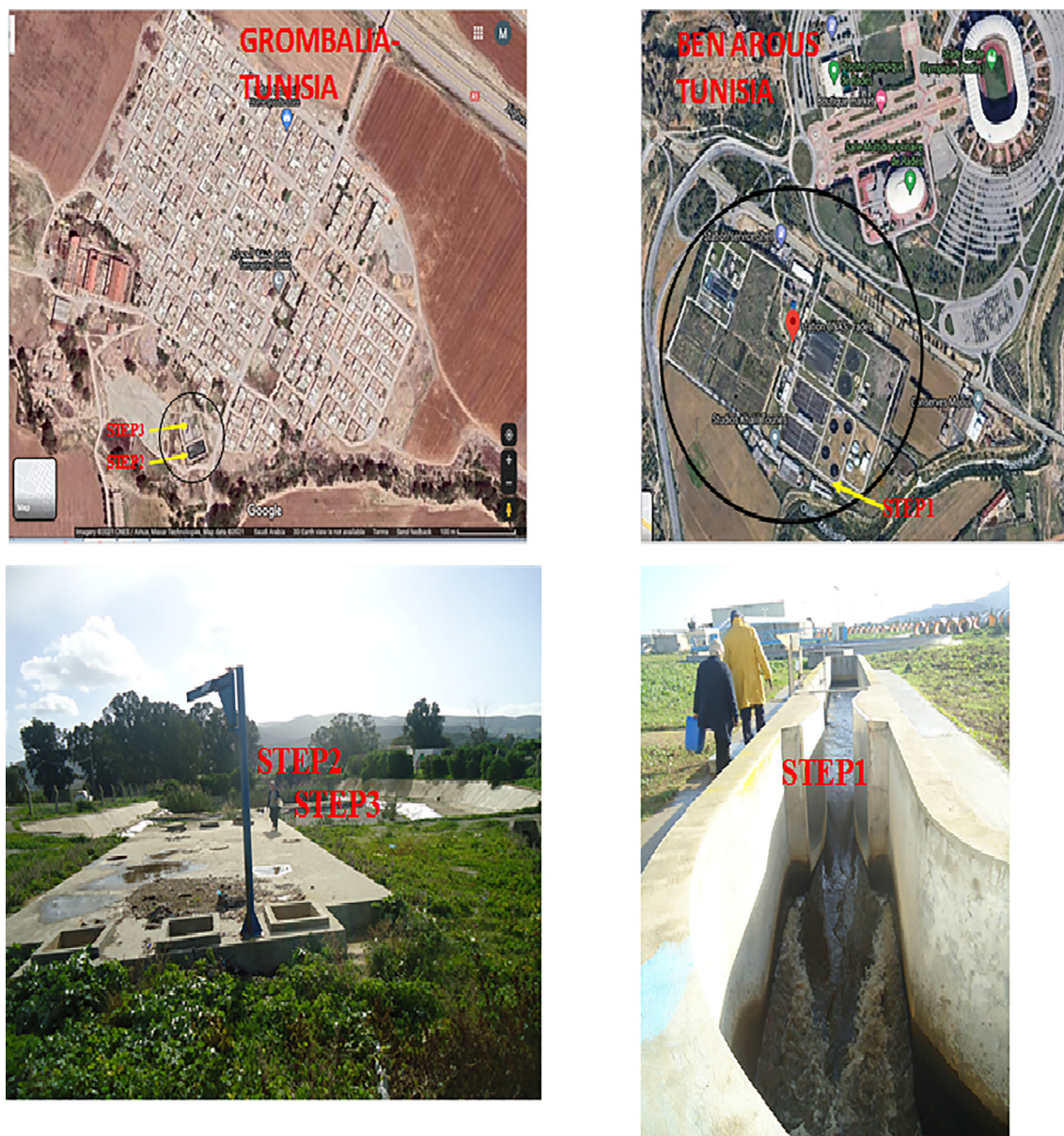
Fig. 2 Wastewaters treatment plant from Rades Malienne secondary treatment (STEP1), Grombalia horizontal treatment (STEP2) and vertical treatment (STEP3).
